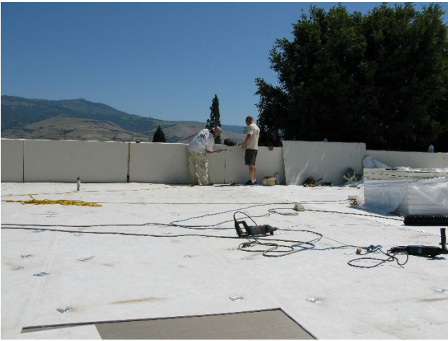
Insulation & Cover Board
