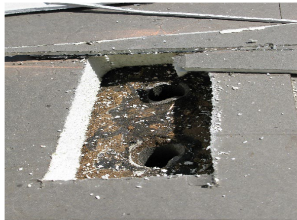
Insulation at Roof Drain
