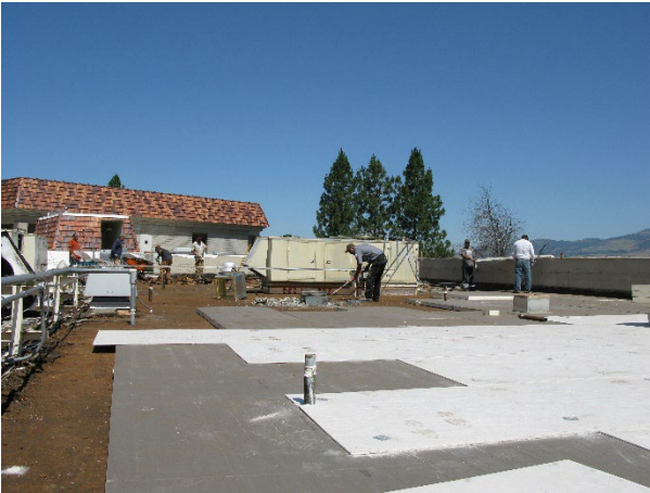
Typical Insulation & Cover Board
