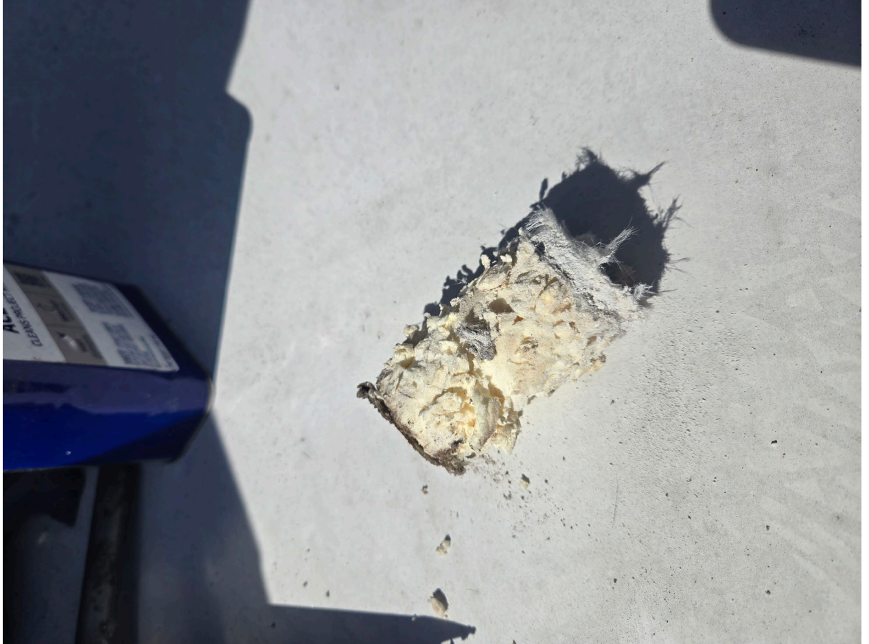
Middle Roof – Photo #1
