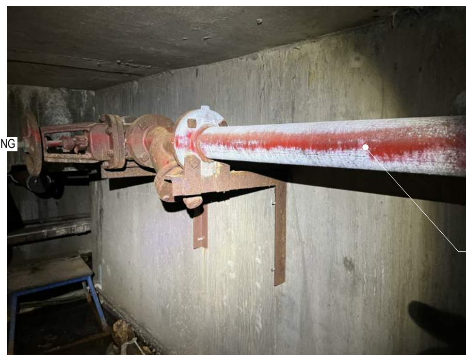
5 LOOKING WEST NEAR LADDER NOT TO SCALE
