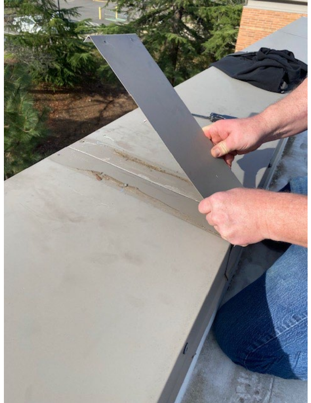
Joint Cover – New Roof
