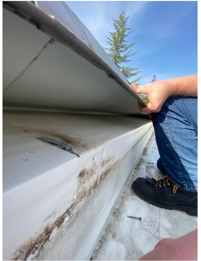
Underside of Coping – New Roof
