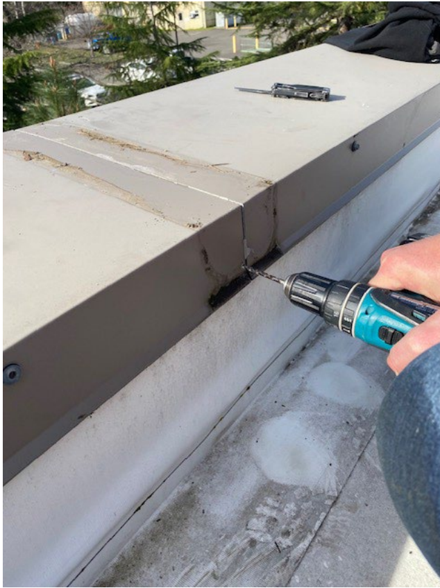
Drilling Backing Plate Rivets – New Roof
