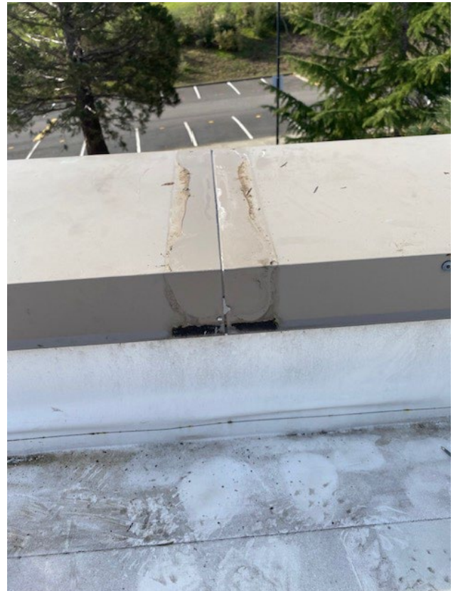
Backing Plate Riveted – New Roof
