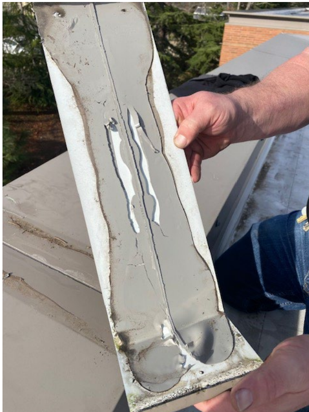
Joint Cover Sealant – New Roof
