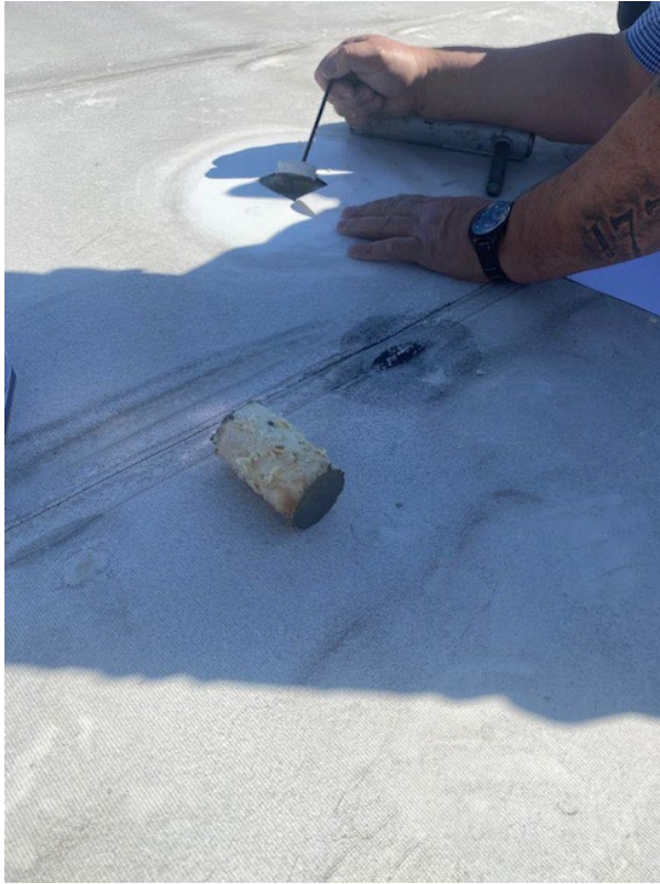
New Roof – Main Section DuroLast over 3" insulation over concrete
