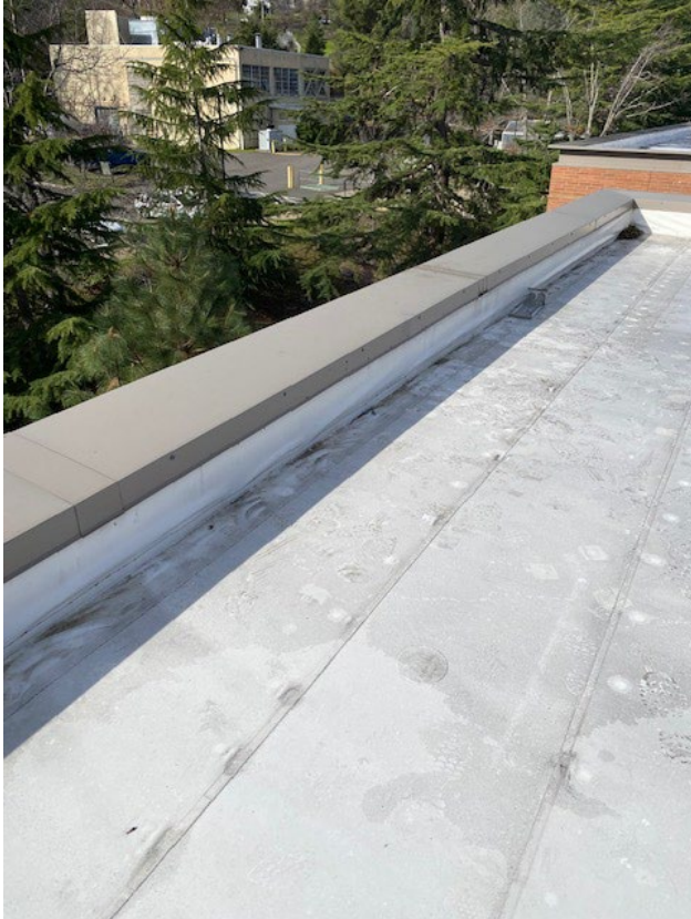
Typical Parapet Coping – New Roof
