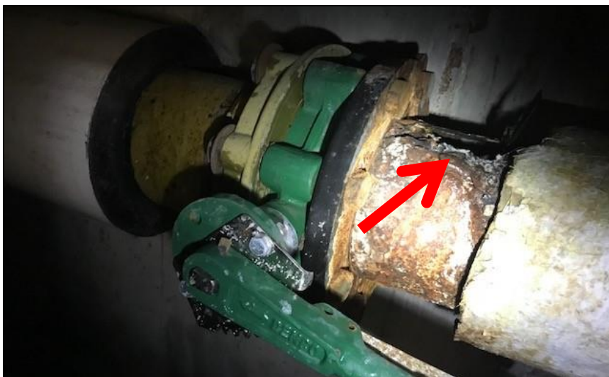
FIGURE 4: RUPTURED PIPE IN TUNNEL
