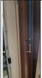
3 typical instances in shop, disconnect stainless tube and lower ball valve and plumb directly to AirNet installed ball valve. Posi-Drain should attach to nearest wall approximately at 42"
