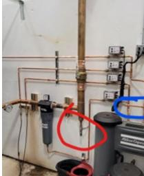
Install in compressor building. Posi-drain can be located low and routed from ball valve to existing 'T' at water/oil separator
