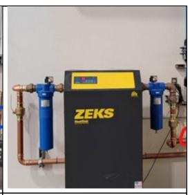
Install at air dryer. Posi-Drain can be installed near existing Posi-Drain and plumbed to oil/water separator. Over extended ¼" pneumatic hose should be extended using either a new line or a stainless union so it is not so tight. Clear hose leading from existing Posi-Drain should be replaced with copper pro-press fittings
