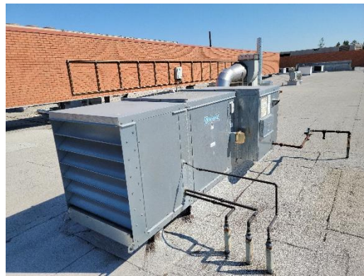
Figure 21: Make-Up Air Unit
