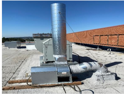
Figure 19: Chemical Storage Exhaust
