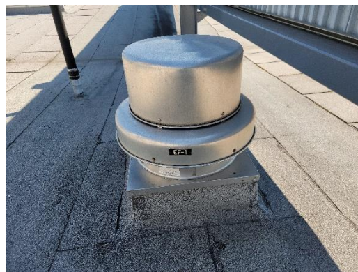
Figure 15: Exhaust Fan
