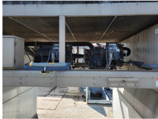
Figure 13: Air Handler (AC-2) Compressors
