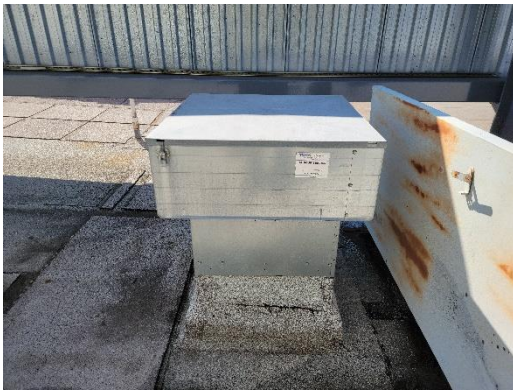
Figure 20: Stair Pressurization Fan
