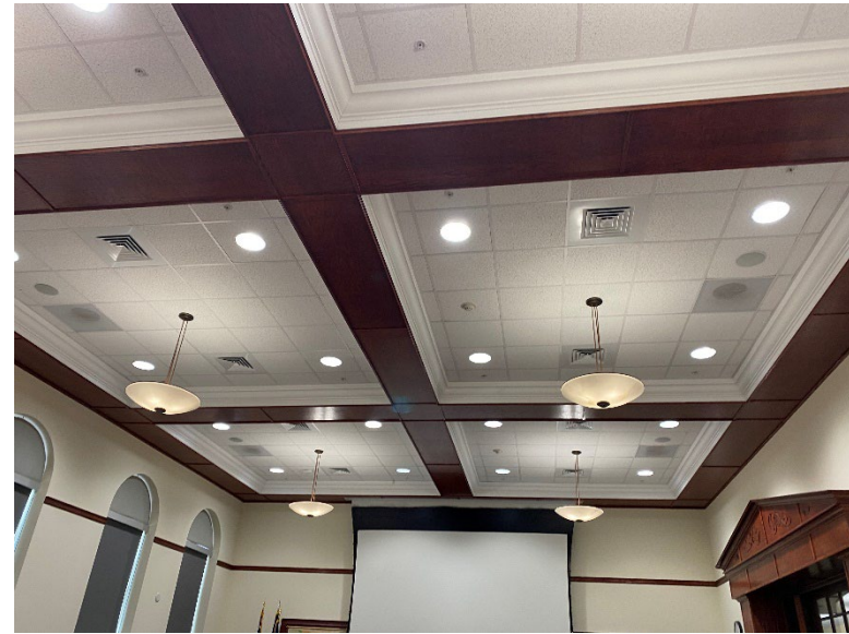
The ceiling is comprised of 2-foot by 2-foot suspended ceiling tile.
