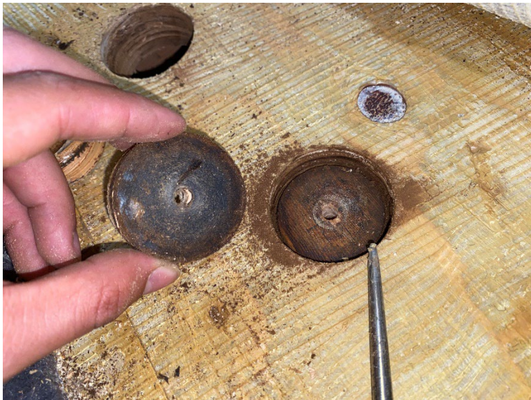
A black tar squeak paper was identified beneath the plywood subfloor.
