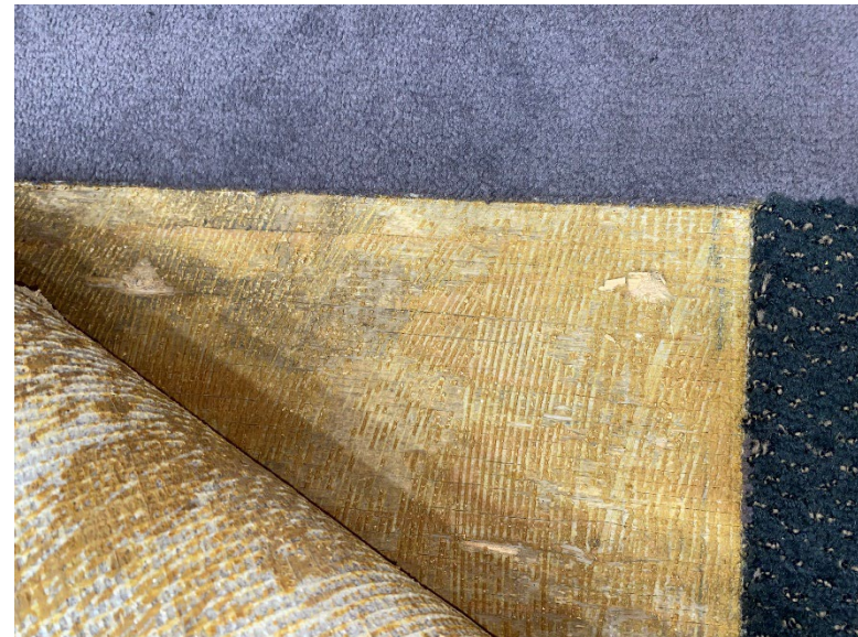
Flooring is comprised of gray and green carpet with tan adhesive on plywood underlayment.
