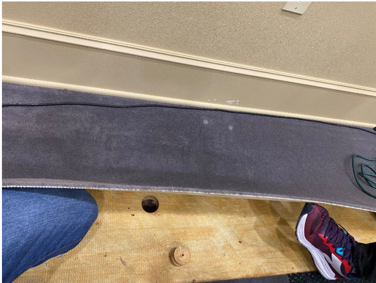
Fulcrum completed drilling of the plywood subfloor.
