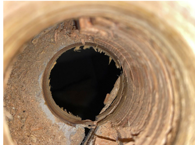
Original wood flooring was observed beneath the plywood subfloor.
