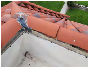
ACM black sealant on metal flashing along perimeter
