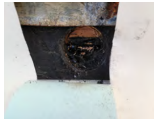
ACM built up roofing on center roof parapet
